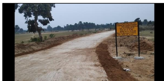
Plate 4: Construction of Roads
